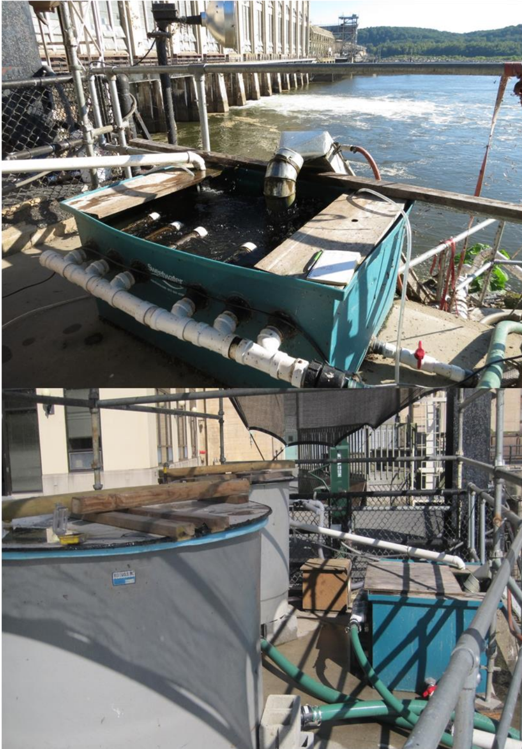
Figure 7. Collection tank and holding tanks located on the lower platform, at the top of the elver ladder, Conowingo Dam, Maryland. Credit: USFWS/MDFWCO/JMalavasi.
